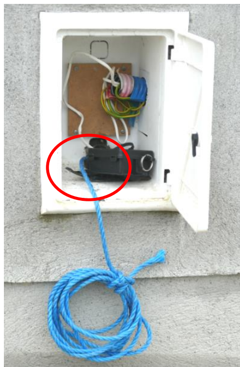
ETU at premises with draw rope installed.
