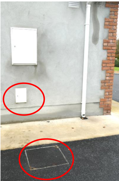
Premises where an access box and ETU are fitted.
