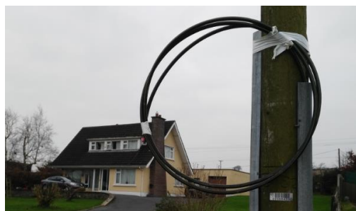
Figure 8 - Transition from underground to overhead - use sub-duct and capping steel
